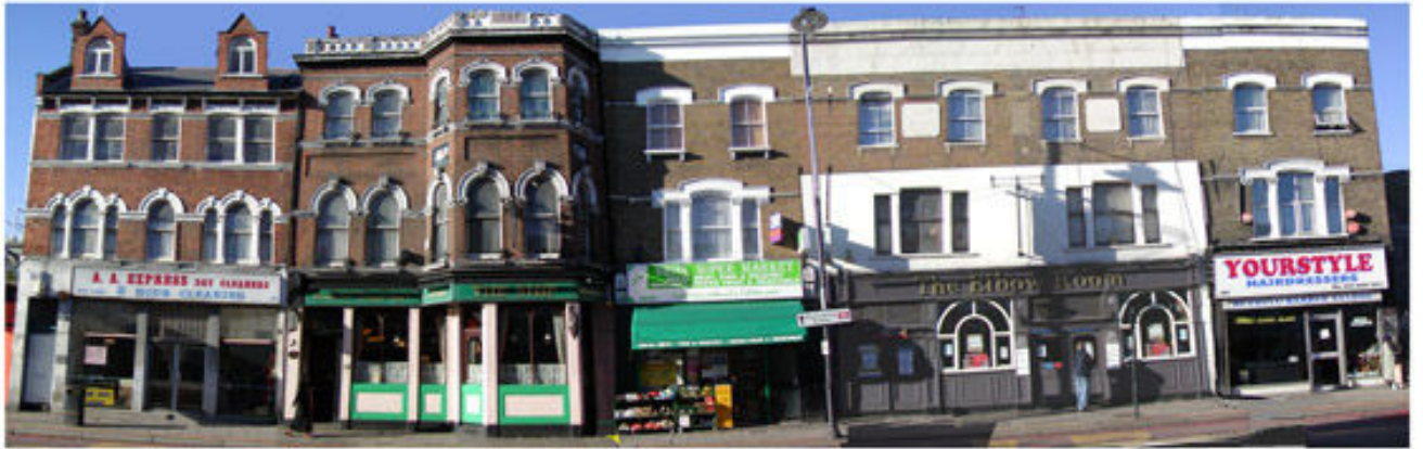
Photograph 1: Elevation of properties – 497-507 Tottenham High Road
